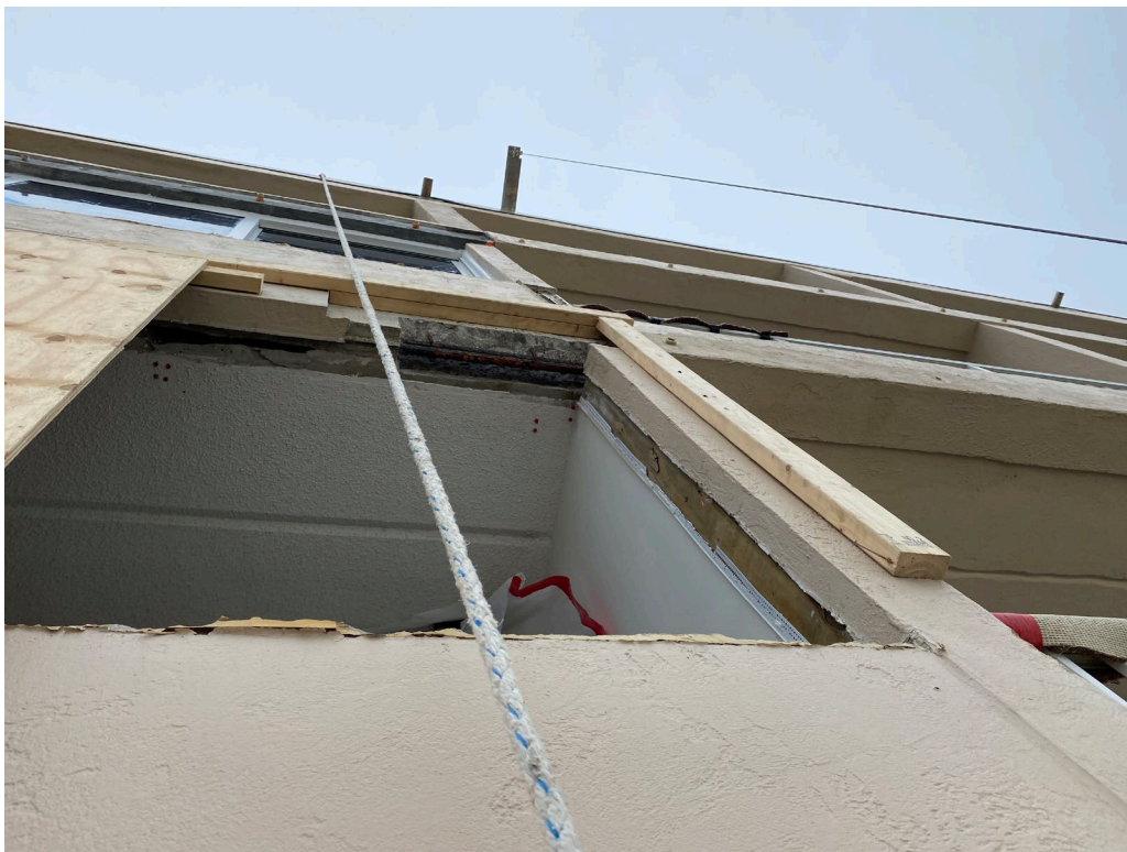
Picture 1: Unit 502 window header repair
