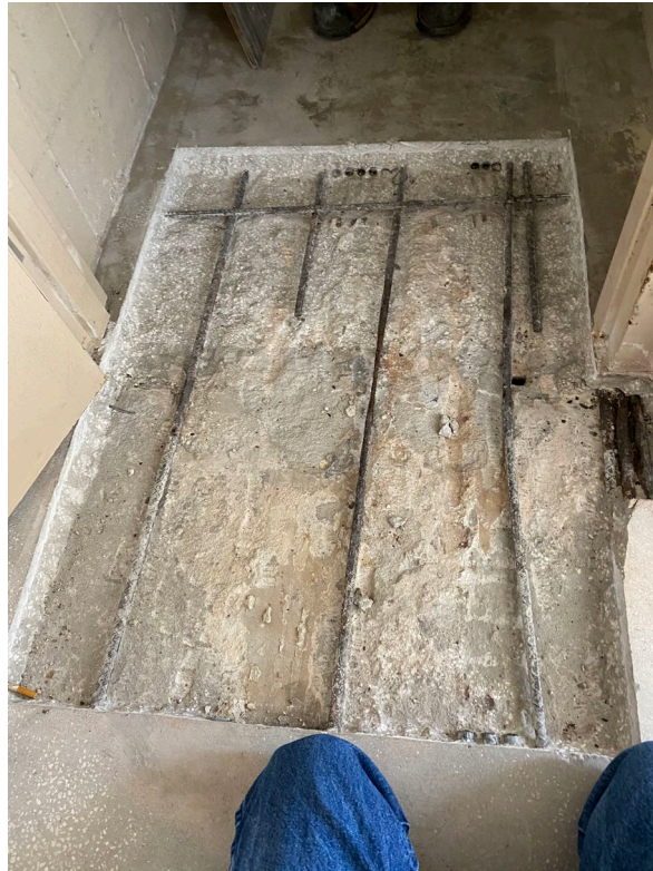
Picture 3: Topside repair at 7 th floor trash room
