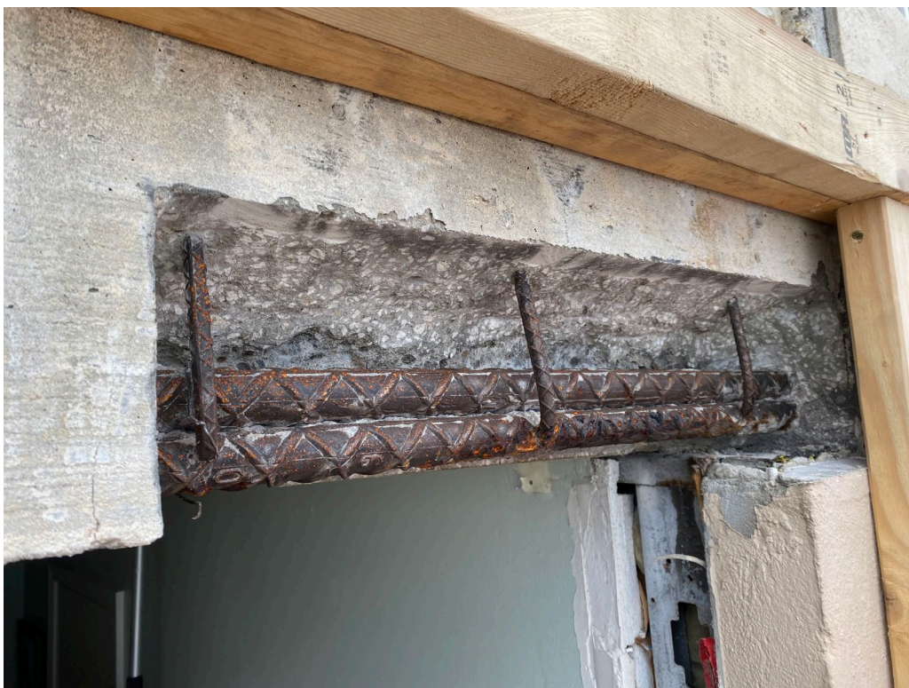
Picture 2: Unit 402 window header repair
